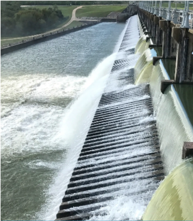
Flood gates at Lake Corpus Christi, May 2019
